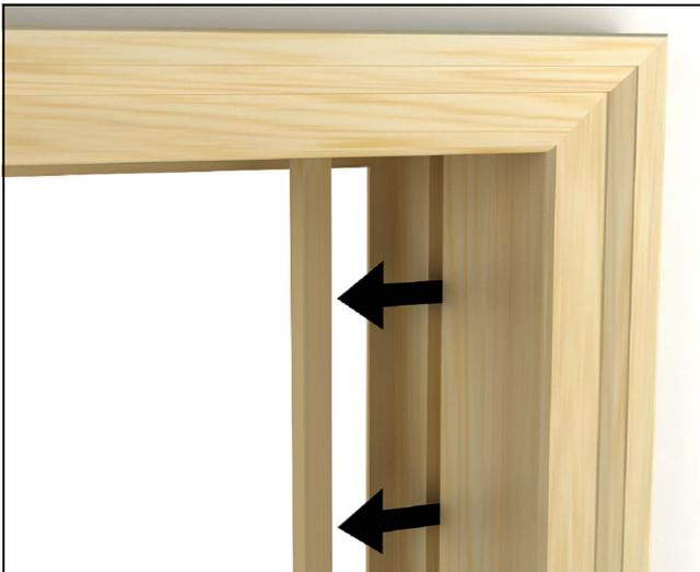
Figure 3 Remove parting stops from side jambs
