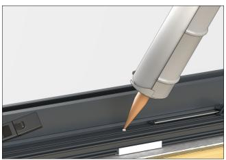
Figure 27 inject installation holes with sealant prior to fastening.
