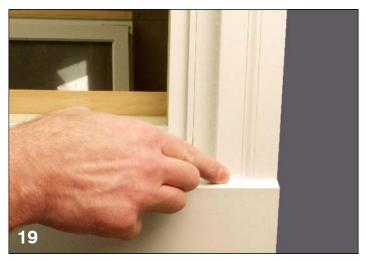
26. Seal the joint between panning and exterior of dwelling with compatible sealant. Be sure to tool out bead of sealant for best performance.
