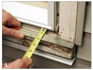
8. Extend these marks at right angles until they intersect. With a hacksaw, cut a notch in the sill panning and remove any burrs with a metal file. Remove an additional 1/16" from the back side of the sill panning. This will allow clearance for the jamb panning. See figure 6. Test fit sill panning to make sure it fits properly around existing jamb casing. Some trimming may be necessary.
