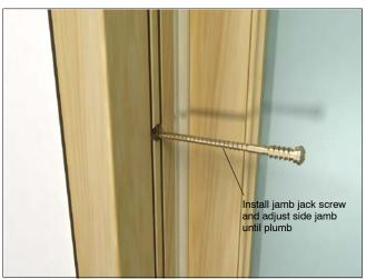
Figure 7: Install jamb jack and plumb jambs
