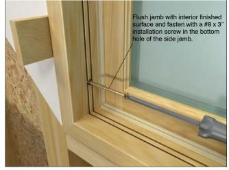
Figure 6: Flush with interior surface and screw through lower end of side jamb
