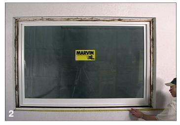
3. Determine the height of the sill panning by using a small sample of the left over component after it has been cut to width. Rip approximately an inch off the face of the component. Set this sample on the insert unit and place an angle finder on the face of the sample. When the sill component is perpendicular to the building, record the height from the bottom of the masonry opening to the front edge of the sill panning sample. See figure 3. Rip the sill panning component to this measurement.
