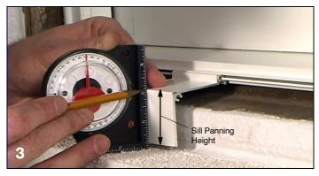
4. Temporarily set the sill panning in the masonry opening against the existing jamb casing. Mark on the sill at the interior edge of the existing casing. See figure 4.
