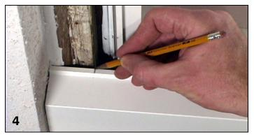
5. Measure the distance from the face of the insert unit to the edge of the sill panning. Add approximately 1/8" and transfer this measurement to the sill panning. Extend these marks at right angles until they intersect. See figure 5.
