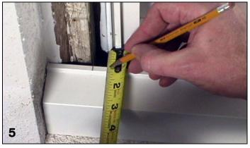
6. Make an additional mark on sill panning at the interior edge of the accessory kerf and over toward the existing jamb casing. This cut will allow clearance for the jamb panning later. See figure 6.
