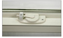
NOTE: The tamper resistant screw cannot be readily removed in case of fire or emergency.
