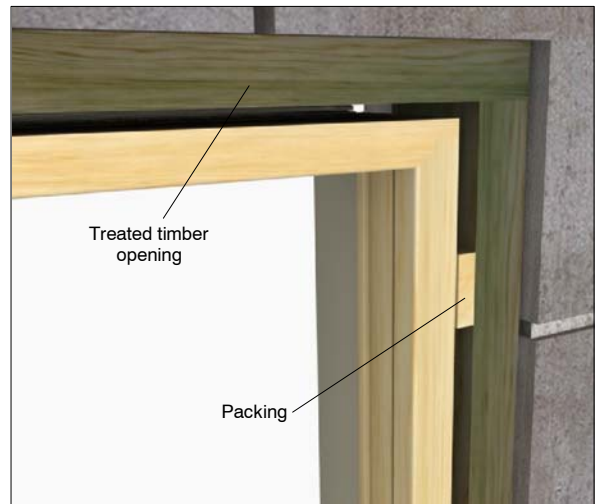
Square the unit; insert packing and fix at the corners
