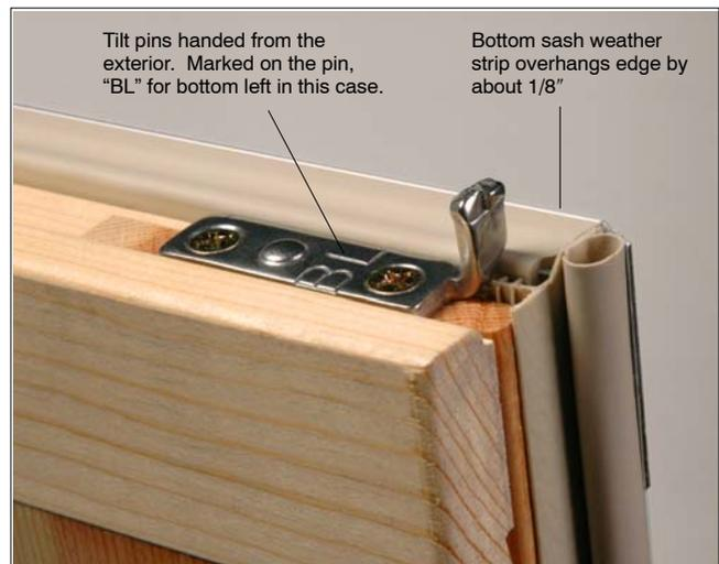
Figure 2: Replacing tilt pins and bottom sash weather strip
