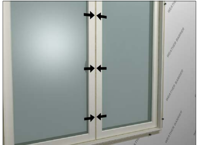
Figure 10: Adjusting the reveal between the sash
