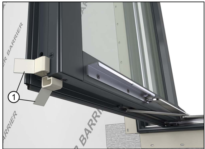
Figure 26 Shipping blocks are located at each corner.
