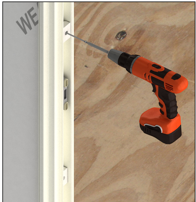
Figure 4 Secure blocks through jambs with 3" screws.
